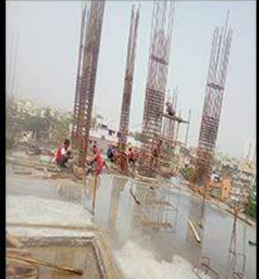
Slab Custing & Column Steel Binding
